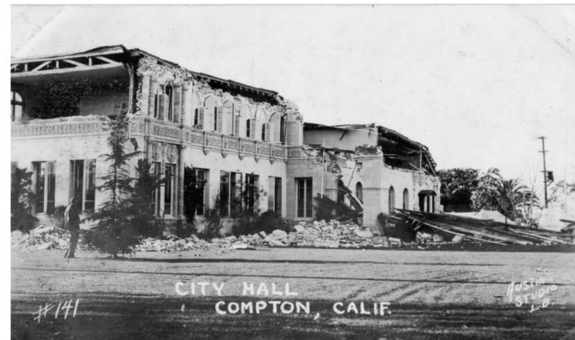
Side view of Compton City Hall shows collapsed walls from 1933 Long Beach Earthquake.
