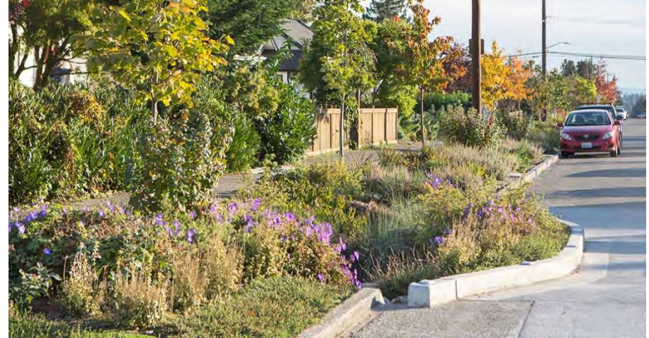
Green Streets use natural processes, including filtration through plants and soil, to treat water runoff in an environmentally friendly way
