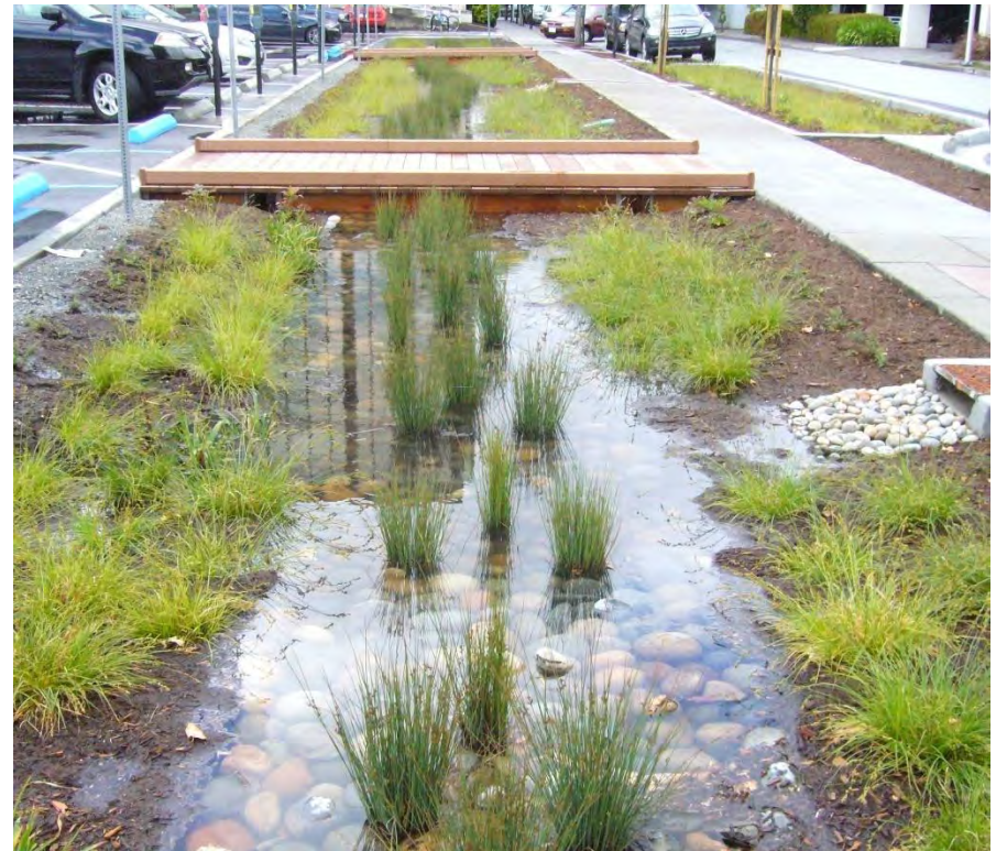
An example of bioswale to clean and filter water and promote groundwater recharge
